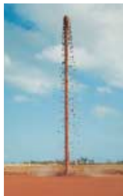
Tower discharge of thickened red mud – ‘dry stacking’ – Alcan Gove, Australia.
